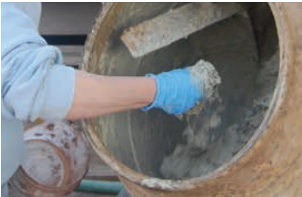
Assessing the workability of the lime hemp plaster and deciding whether or not to add water
