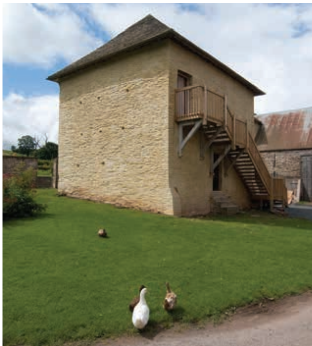
Tŷ-Mawr Training Centre - plastered internally with lime hemp plaster.
